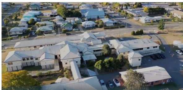
Figure 4: Aerial view of Laidley Hospital
