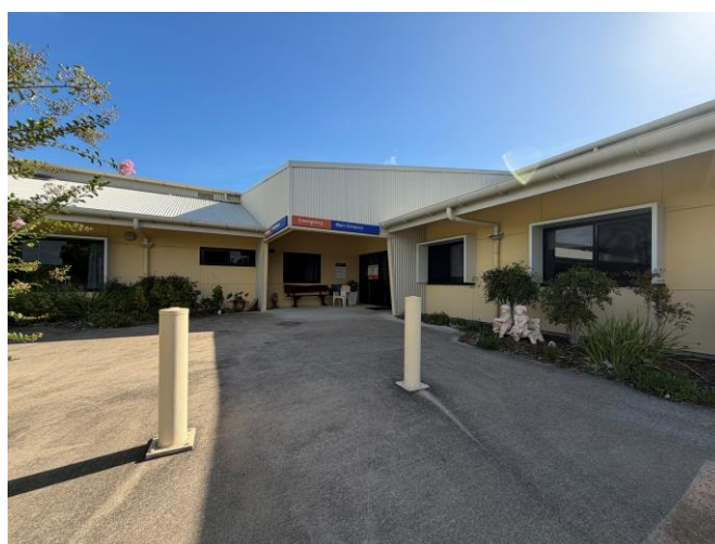
Figure 3: Main Hospital entrance
