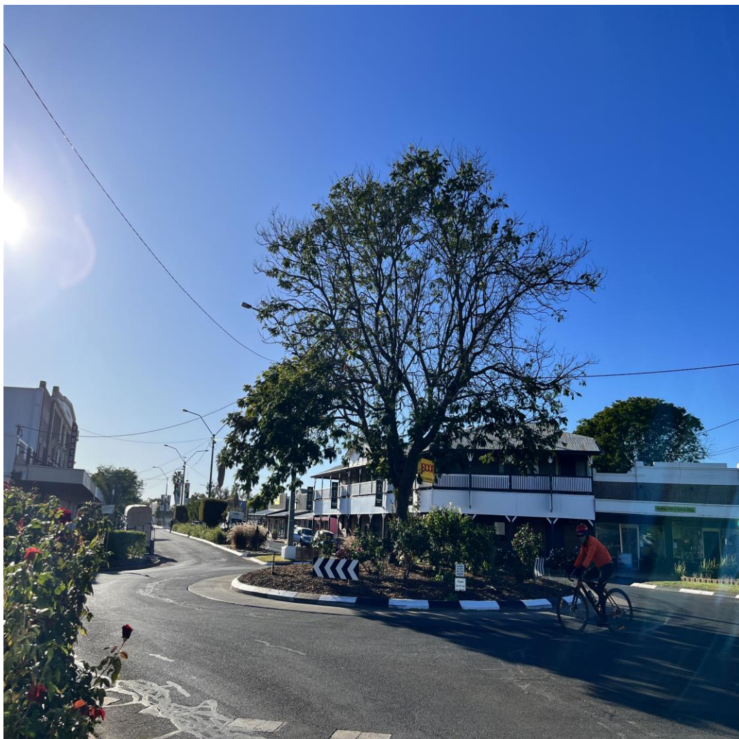
Figure 1: Roundabout in central Cunnamulla at the junction of Jane St, John St and Emma St
