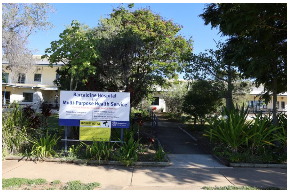
Figure 1: Barcaldine Hospital and Multi-purpose Health Service
