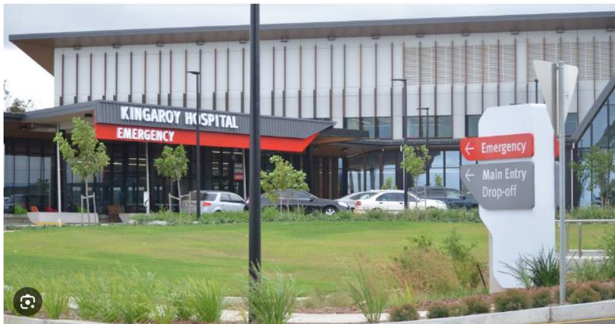
Figure 2: Kingaroy Hospital 166 Youngman Street, Kingaroy, QLD 4610 - new Hospital building completed 2022
